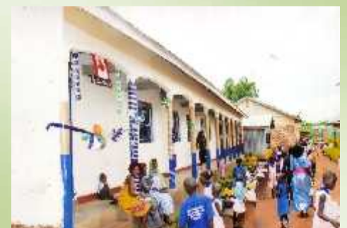
To permanent Blocks
