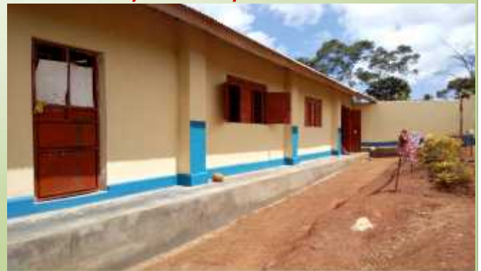
New Boys dormitory Commissioned too
